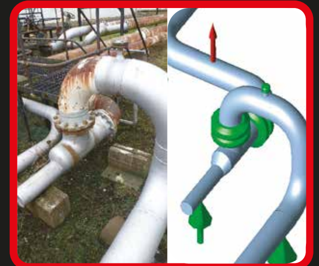
In-situ live lift stress analysis for Corrosion Under Insulation on Pipeline
