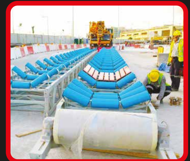
Rollers and Pulley Replacement
