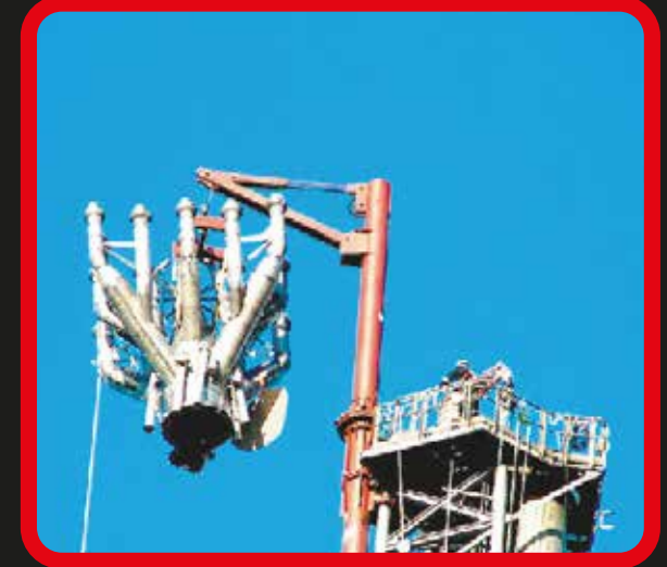
Davit System for Tip Replacement
