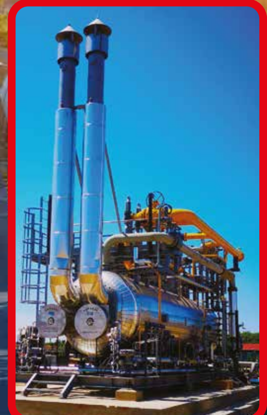
Waster Heat Recovery Boiler
