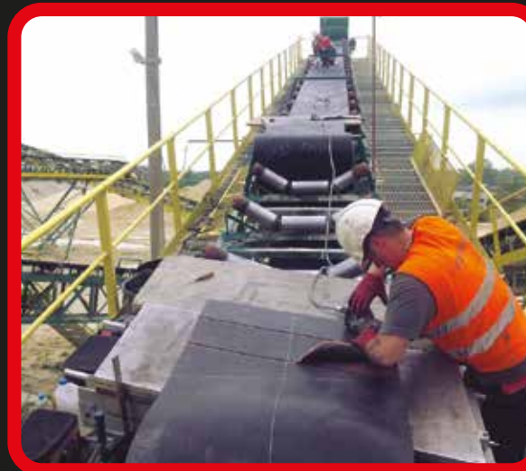
Conveyor Belt Repair
