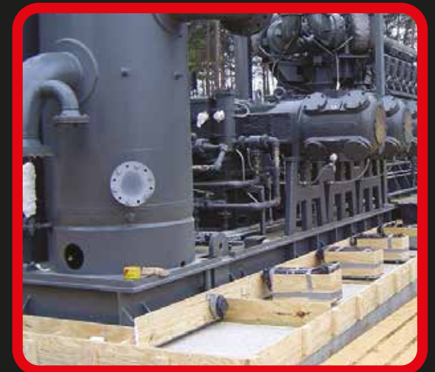
Epoxy Grouting
