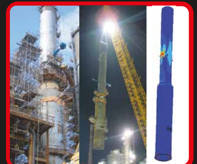
400 T PV decommissioning for top and tail lift, including initial damage and Fitness for Service
