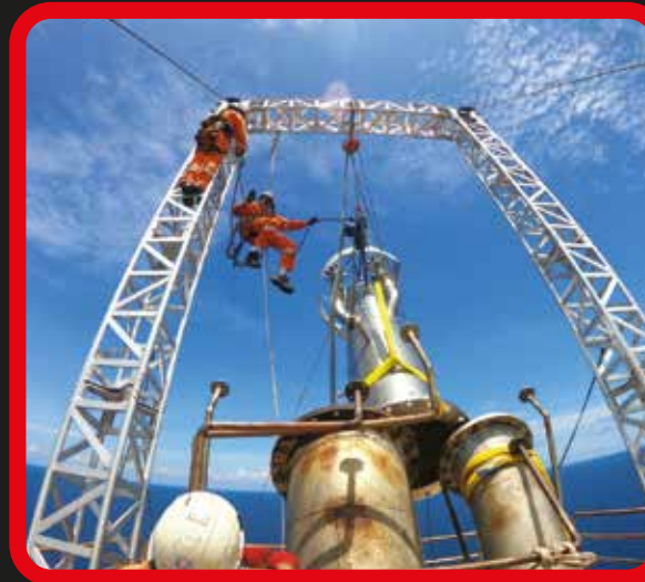
Offshore Flare Tip Replacement
